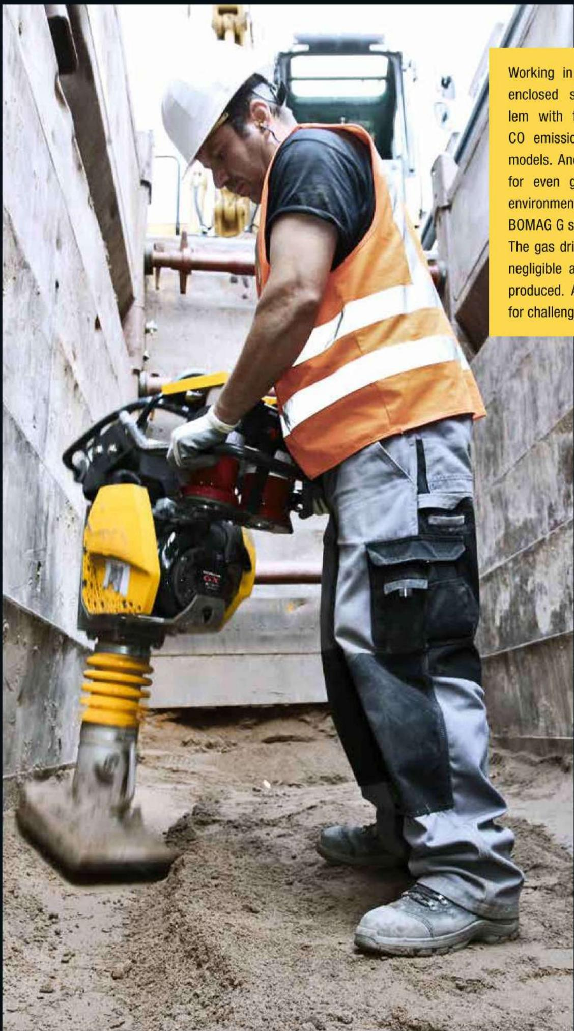
Working in deep trenches or enclosed spaces? No problem with the new reduced-CO emission BOMAG tamper models. And for users wishing for even greater safety and environmental features, the BOMAG G series is the answer. The gas drive unit means only negligible amounts of CO are produced. A practical solution for challenging job conditions.
